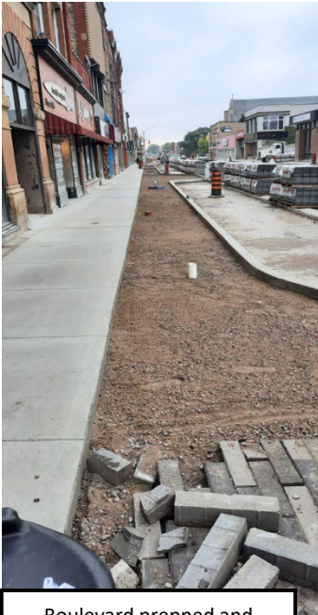
Boulevard prepped and ready for brick pavers
