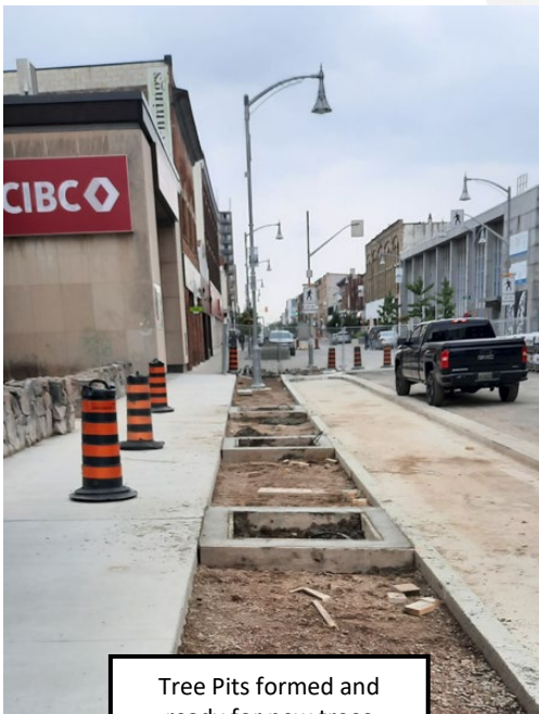
Boulevard prepped and ready for brick pavers
